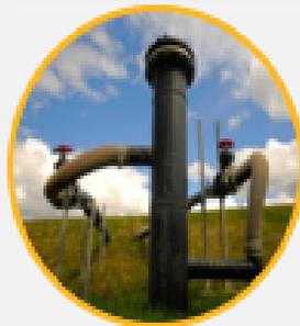
Wells are drilled at the landfill for landfill gas collection and are put under vacuum for central collection
