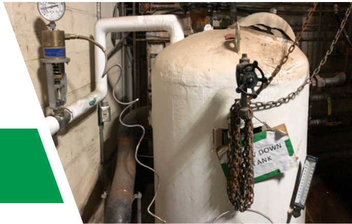
(image on the left) from Credit Valley Hospital Case Study: Blowdown tank, municipal water line, and temperature regulating valve that previously cooled boiler blowdown water before it went to the drain. (image on the right) from Arla Foods Case Study: Component of CIP system.
