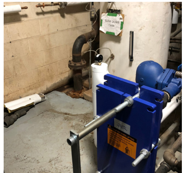
Image from Credit Valley Hospital Case Study: View of new heat exchanger (blue object in foreground) and previous blowdown cooling system in background.
