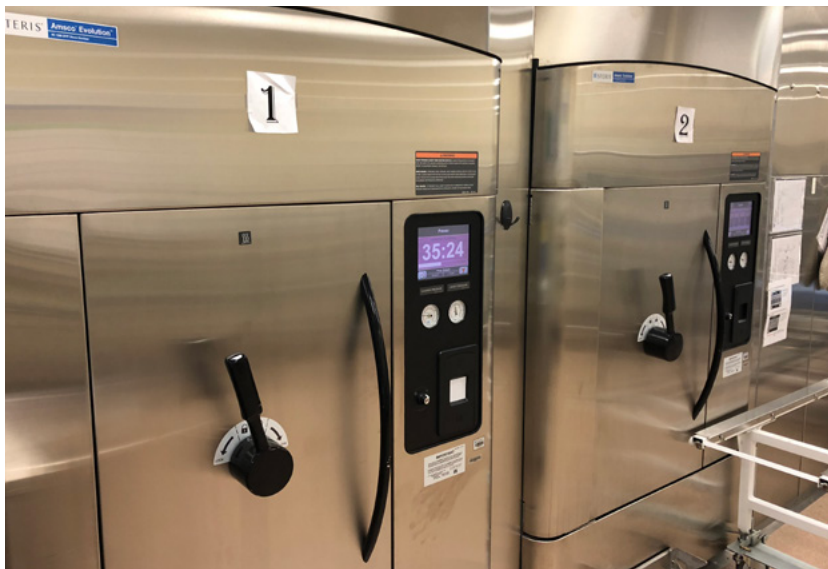
Image from Credit Valley Hospital Case Study: Front view of two new steam sterilizers.
