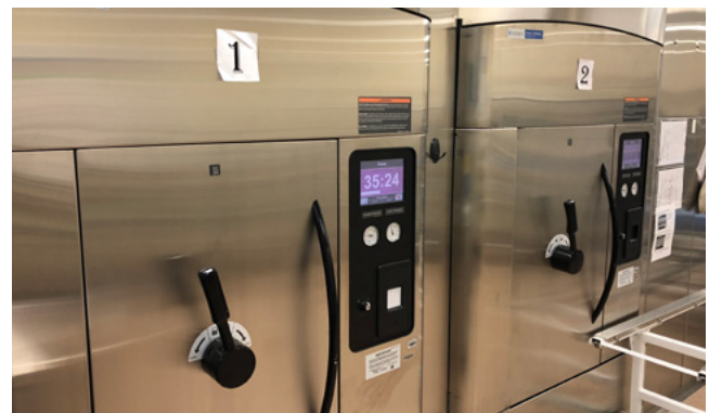
Front view of two new steam sterilizers.
