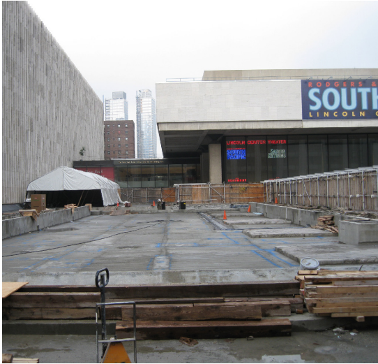
The North Plaza prior to installation
