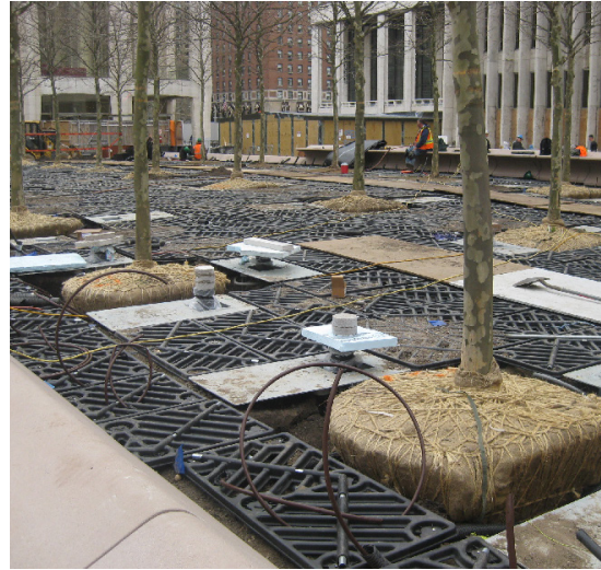
Custom metal decks were used around the tree openings to make the lights work in the thinner paving.
