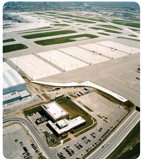
Toronto Pearson's Central Deicing Facility - at the time of construction was the largest in the world.
