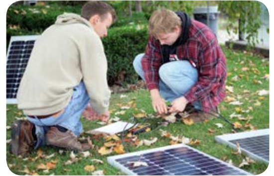
Solar panels provide energy to the grid, which has incentives through the FIT program
