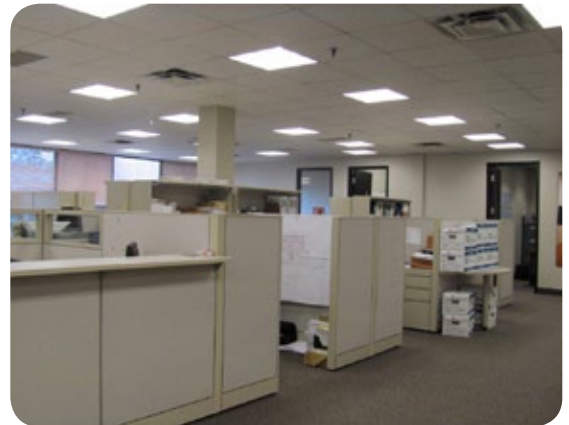
Cooper's office lighting retrofit saves the company money on hydro bills while providing an improved lighting environment for staff
