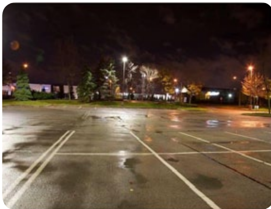
Switching to LED fixtures in Cooper's parking lot reduced energy consumption by about 50 per cent and hydro costs by about 60 per cent
