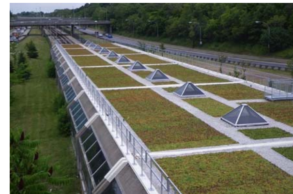
Toronto Transit Commission's subway system – Eglinton West station boasts a 790 m 2 green roof. (Credit: Gardens in the Sky)
