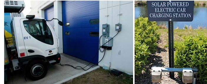
Solar-powered electrical car charging station and Electric Delivery Trucks. (Credit: Testa Produce Inc.)
