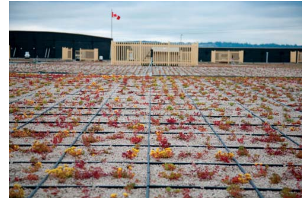
A green roof being planted on a Walmart Supercentre in Port Coquitlam, BC. (Credit: Onni Group)
