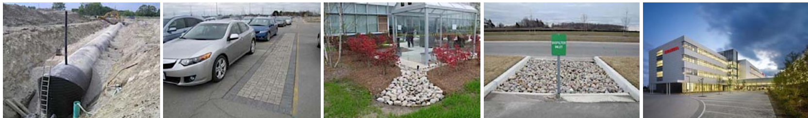
Photo (Left to Right): Underground rainwater harvesting tank; permeable pavement at parking lot; natural drainage; biofilter inlet; permeable pavement in Forecourt roundabout (Credit: Schollen & Company Inc.)
