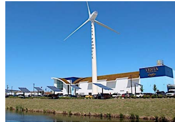
A wind turbine and solar panels are mounted in the Testa Produce's refrigerated storage facility in Chicago. (Credit: Nick Przybyciel/MEDILL)
