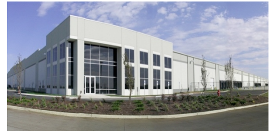
Figure 30. Kellogg's Distribution Centre, West Jefferson, OH (Credit: ALD Precast)
