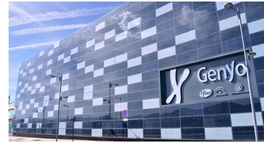
Figure 48. Building Integrated Photovoltaics. (Centre for Genomic and Oncologic Research Centre (GenYo), Spain. Credit: Onyx Solar)
