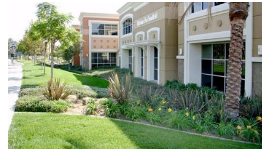
Figure 32. Landscape Setbacks. (Shelby Office Park, California. Credit: Ridge Landscape Architects)
