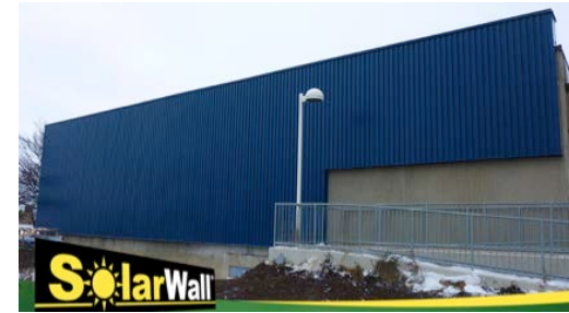
Figure 49. Solar wall installed at Mayfield Recreation Centre, Caledon. (Credit: Conserval Engineering Inc.)
