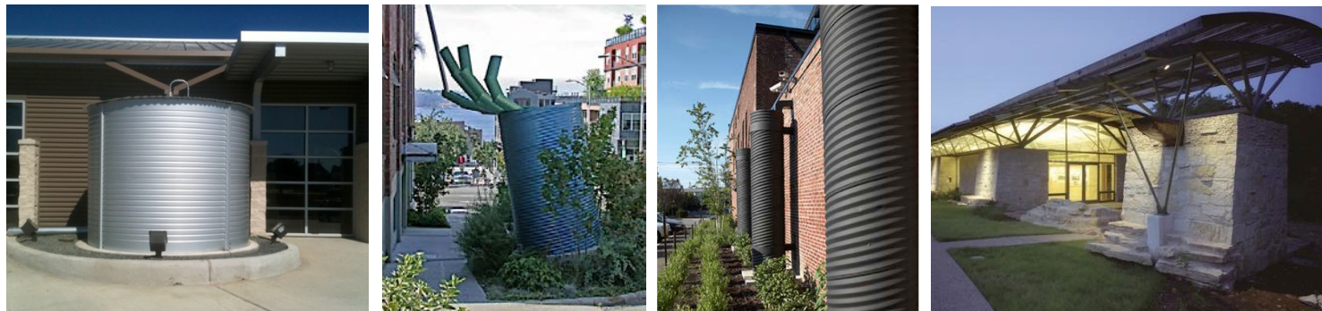
Figure 43. Rainwater Cisterns collect and store rainwater for re-use. Right: Warren Skaaren Learning Center, Credit: Greg Hursley
