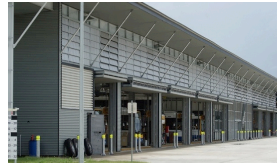
Figure 52. Use louvers and circulating fans to provide natural ventilation. (Credit: Austral Monsoon Building Products)
