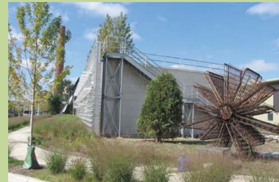
Figure 70. Chicago Green Permit Program. This building features a green roof, permeable pavers and bioswales, which meet Chicago's stormwater management requirements.
