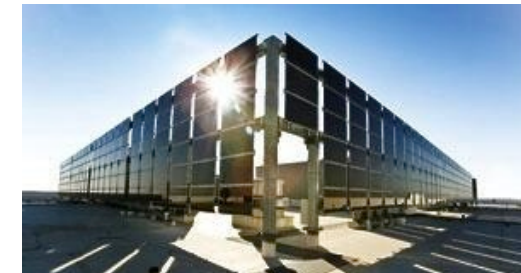
Figure 36. Rooftop Photovoltaic panels/HVAC screen at Modesto Medical Center, CA. (Credit: Kaiser Permanente)
