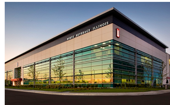
Figure 31. Wirtz Beverage Distribution Centre, Cicero, Illinois (Credit: Ryan Companies US)
