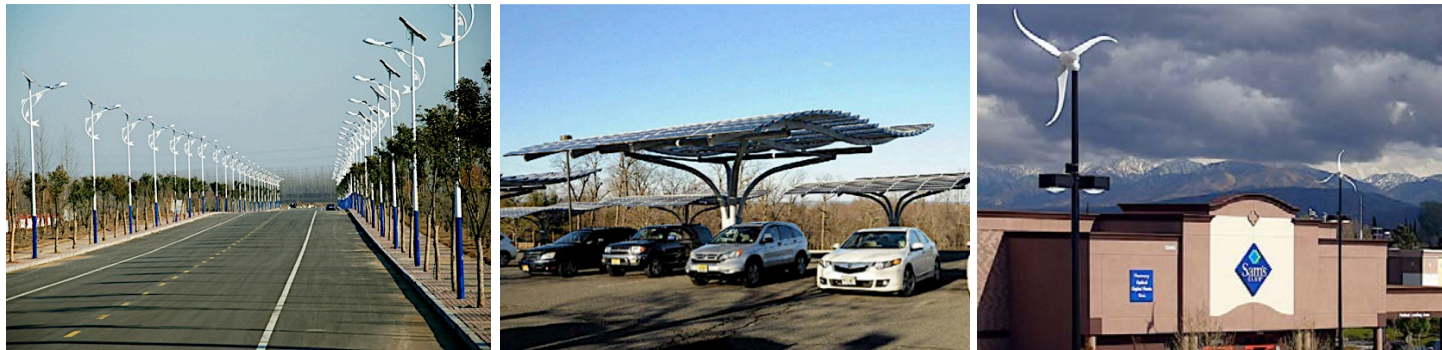
Figure 25. High efficiency outdoor lighting fixtures can also incorporate small PVs and micro wind turbines.
