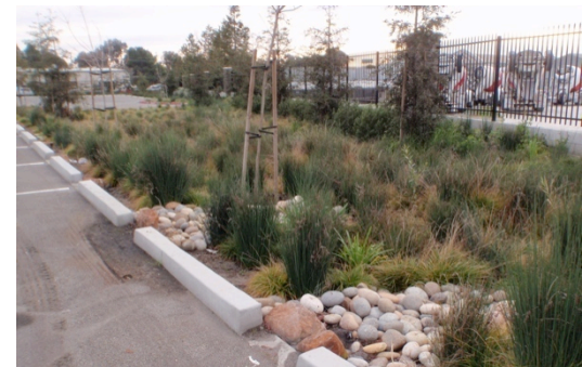
Figure 33. Rain Garden along lot edge. (Lowe's store, Concord, Credit: Blue-Green Building website)
