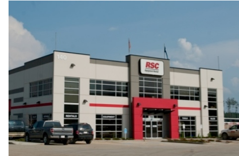
Figure 37. Clearly Marked Site Access. (TaigaNova EIP, AB)
