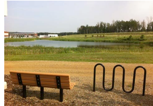
Figure 16. Integrate Stormwater ponds with Open Space Amenities (TaigaNova EIP, AB)
