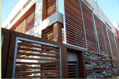
Figure 53. Trombe Wall can be energy efficient and aesthetic appeal. (Credit: Jeremy Levine Design)
