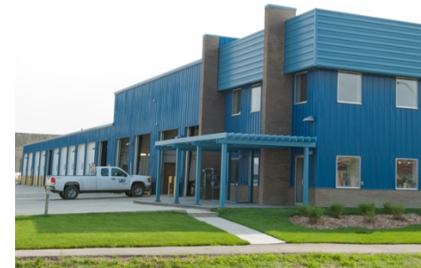
Figure 38. Weather Protection for Pedestrians. (TaigaNova EIP)
